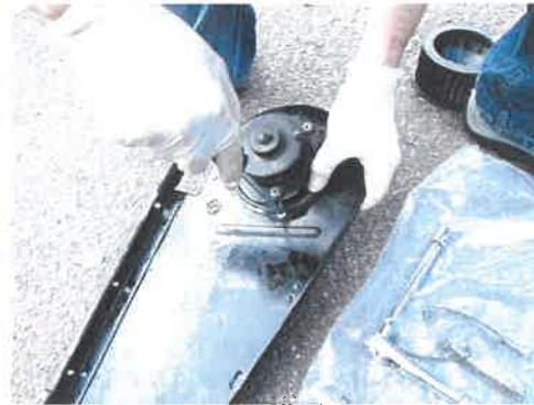
Strip down original system
