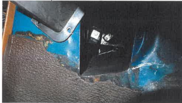
Check Air Control Flap Operation
